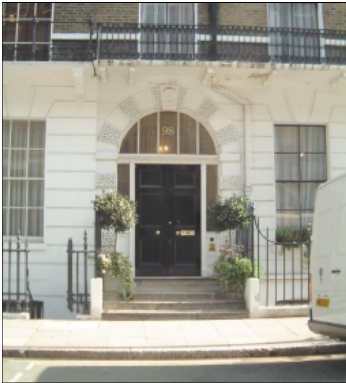
Figure 2: 98 Harley Street. Michael's suite is located on the second floor of the building
